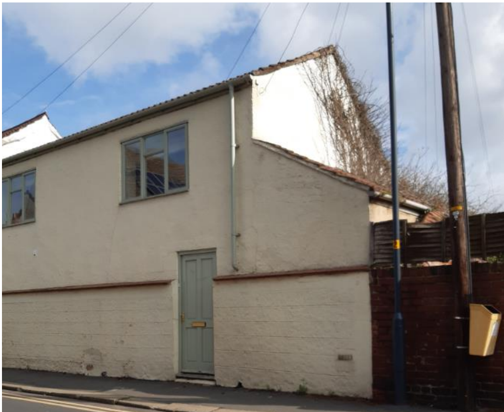
View of the south elevation looking north from Thorpe Lane
